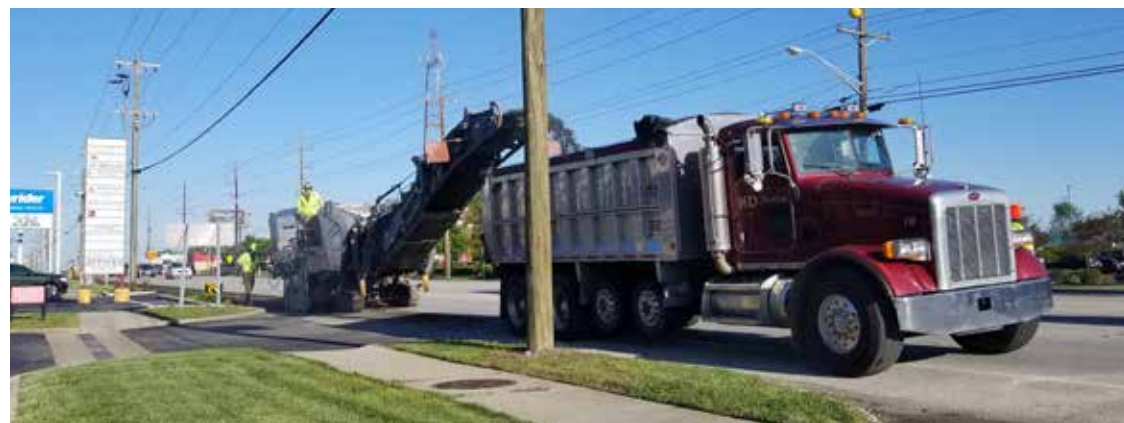
Beechmont Avenue was repaved and restriped this summer.
