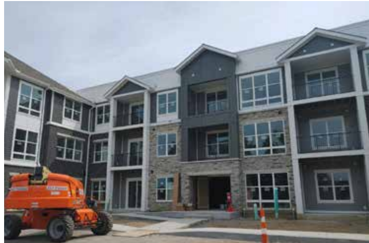
More diverse new housing is one of the goals of the 2016 Comprehensive Plan; pictured is new construction of Stonegate Apartments Phase 3.
