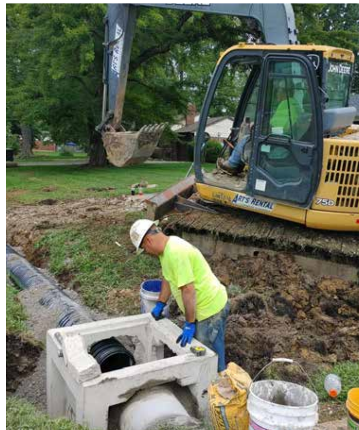
Work on a Nordyke Road sidewalk link began in late summer.
